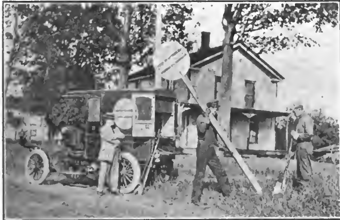
The Completed Post Ready for Erection
